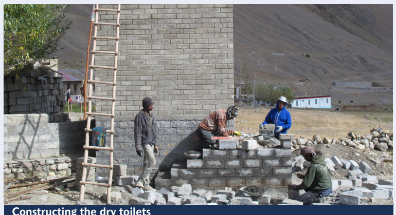
Constructing the dry toilets
