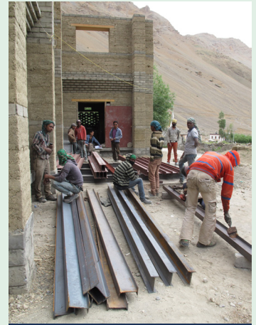
Preparing the steel joists
